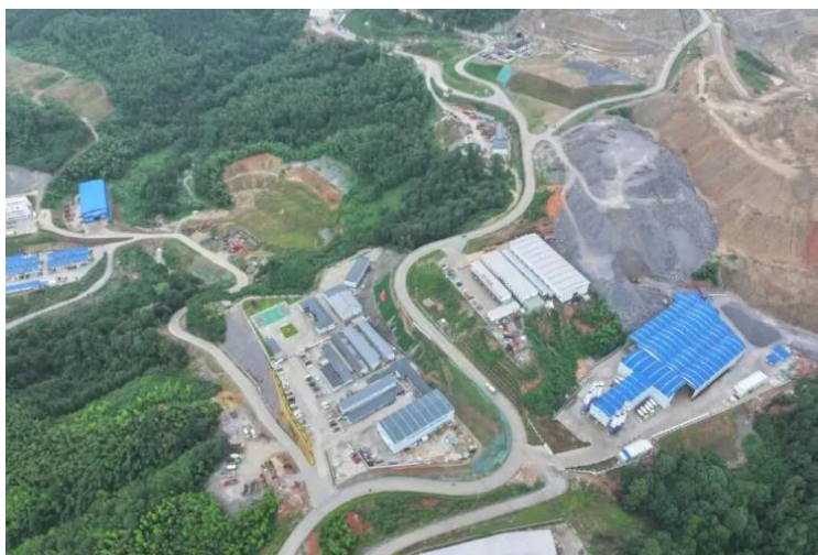
(奉新抽水蓄能电站项目地形概貌)
